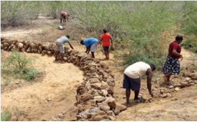
Figure 2.20: Construction of a dike in the Quilombola community Poço do Cavalo (left); Transport of stones for the construction of a dike (right) São Francisco River Basin, Brazil. (Pierson Barretto)
