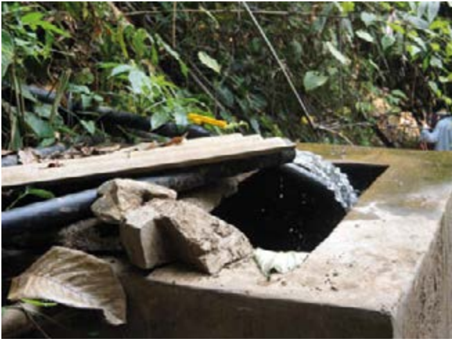
Figure 2.34: Collection point for surface water: the common way to secure water supply for villages, China. (SURUMER)
