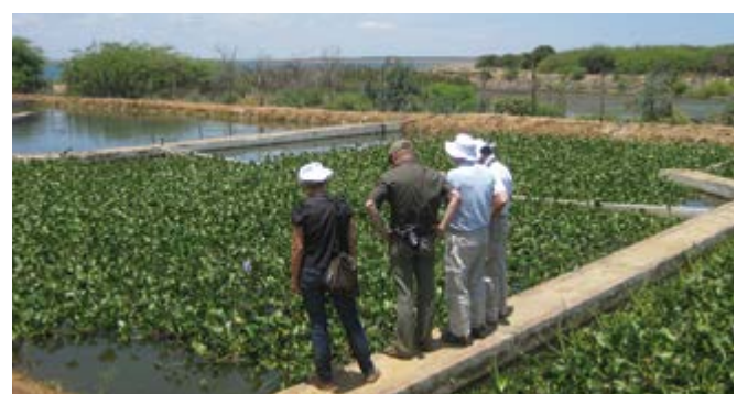
Figure 2.24: Green Liver System for treating aquaculture effluent, Brazil. (Johann Köppel)
