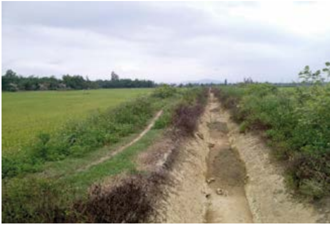
Figure 1.40: Tu Cau irrigation canal stops working due to salt intrusion impacts in Vietnam (March 2013). (Tran Thi Ha Van)
